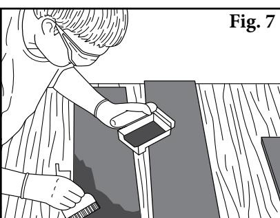
7. **Apply a second coat of adhesive to one strip of lagging.** Be sure to apply adhesive to the edges of the lagging as well.
